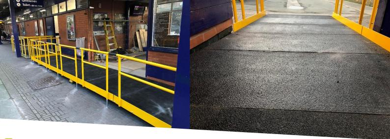
END RESULT: A Rapid Ramp with a slip-resistant GRP surface and yellow 'warm-to-touch' handrails was installed and fully completed within a day.
