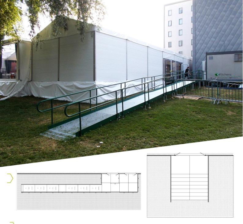
**END RESULT:** A temporary disabled ramp and step unit were quickly designed, selected, packaged, and transported to the site, ready for their installation team to assemble.
